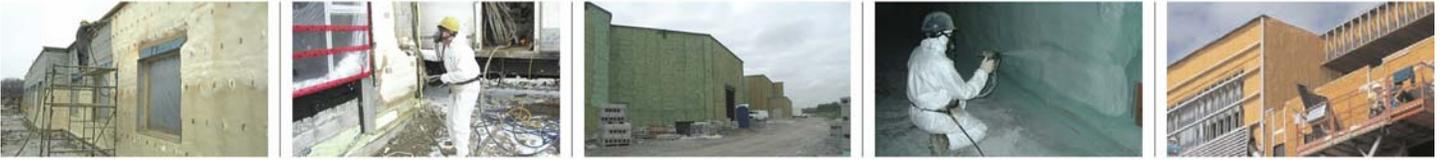
SPF which is 600 mm thick will have a greater RSI per 25 mm when compared to a 25 mm specimen sprayed at the same time as it takes time for this process to move through the material.
